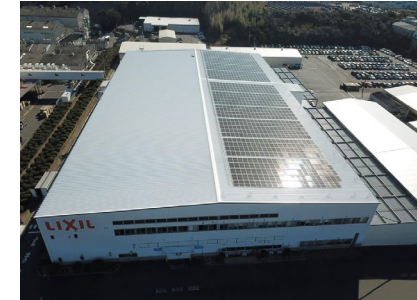
Solar power generation installation
